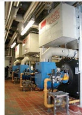
University College London have installed an innovative new boiler plant in it's Torrington Place Building. The boiler house operates throughout the year at 95°C flow and 75°C return, and contributes to the UCL ring main that serves scores of buildings, large and small.
